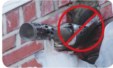
• **Check if the boiler ventilation pipe is dented**
