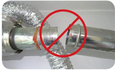
• **Check if the boiler ventilation hood is out of place**
